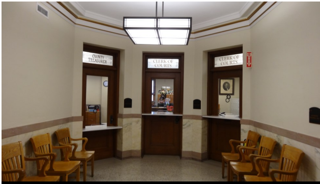
Existing doors were reused as transaction windows in the newly remodeled Clerk of Courts Office.
